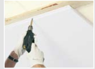
Focus F is installed by screw fixing black
