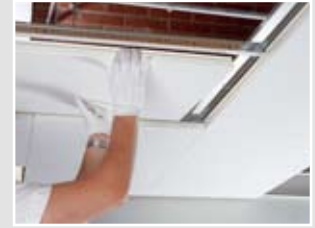
Master Ds, the individual tiles are easily demountable
