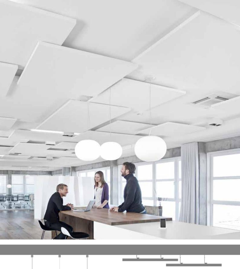
Connect Adjustable wire-hangers allows flexibility in ceiling height and Connect Absorber Anchor makes mulitilevel installation possible.
